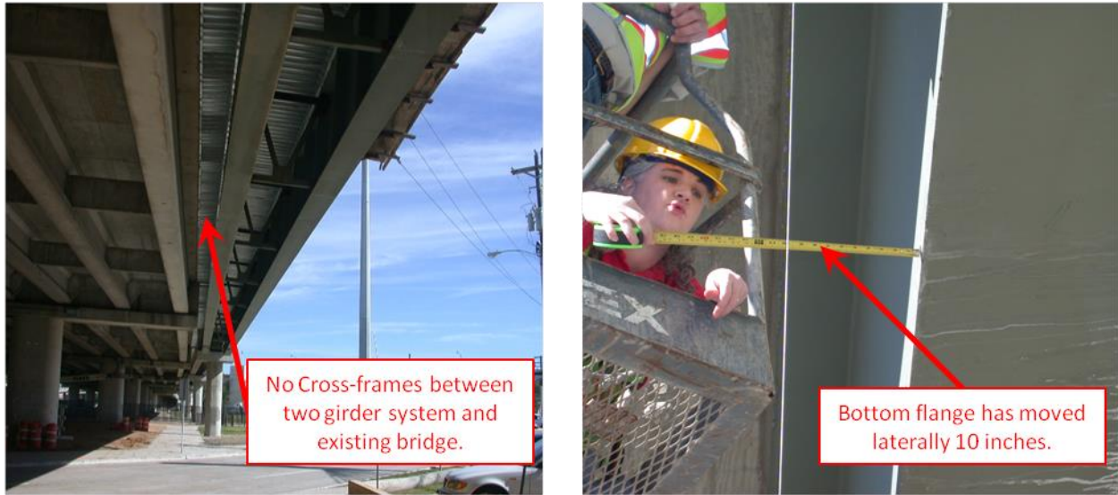
a) Twin Girder Widening
