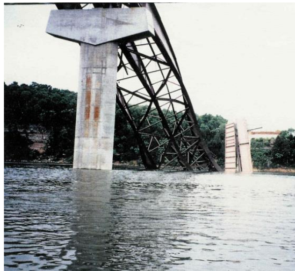
Figure 4 Collapse of a Bridge over the Tennessee River due to Insufficient Bracing
