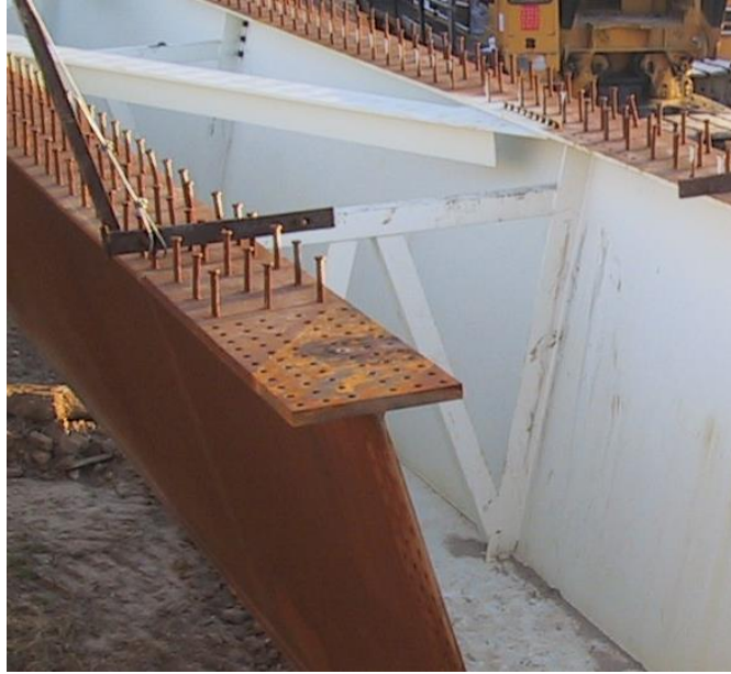
Figure 59 Strut offset below diagonal
